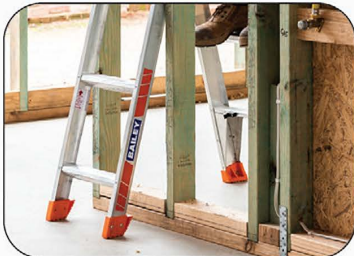
Back legs through studs
