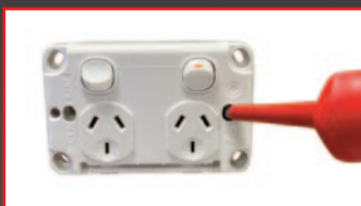
Screw outlet to the quick fit box
