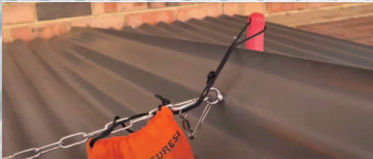
holds roof sheet back for safe access
