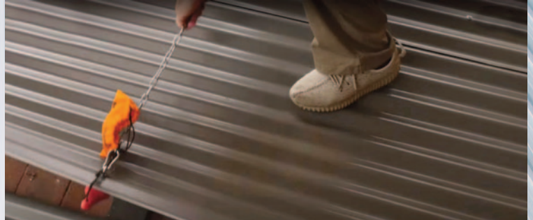
Safely peel back metal roof sheeting
